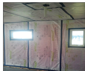
Air tightness/moisture control membrane
